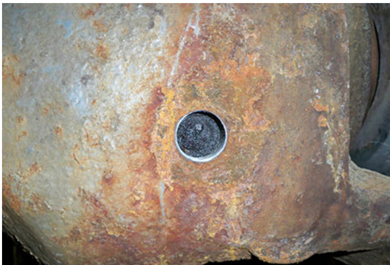
The result of a poorly maintained pump. The bearing frame is full of potash.
