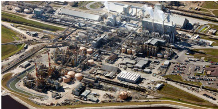
Typical Phosphoric Acid Plant
